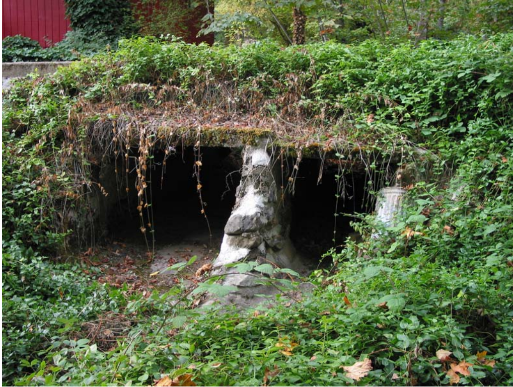
Figure 33. Culvert #10 outlet on Alder Creek at driveway off Canyonville-Riddle Road.
