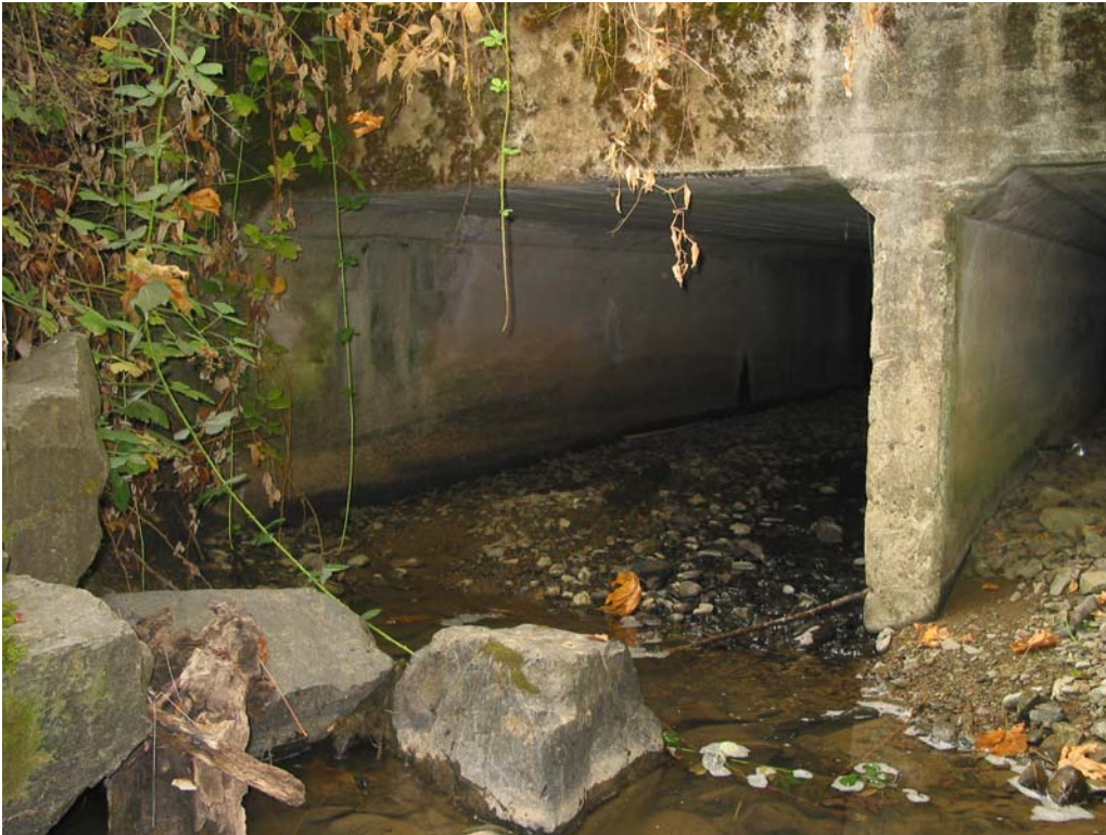
Figure 22. Culvert #1 outlet on Jordan Creek at I-5 (south half of twin box culverts).
