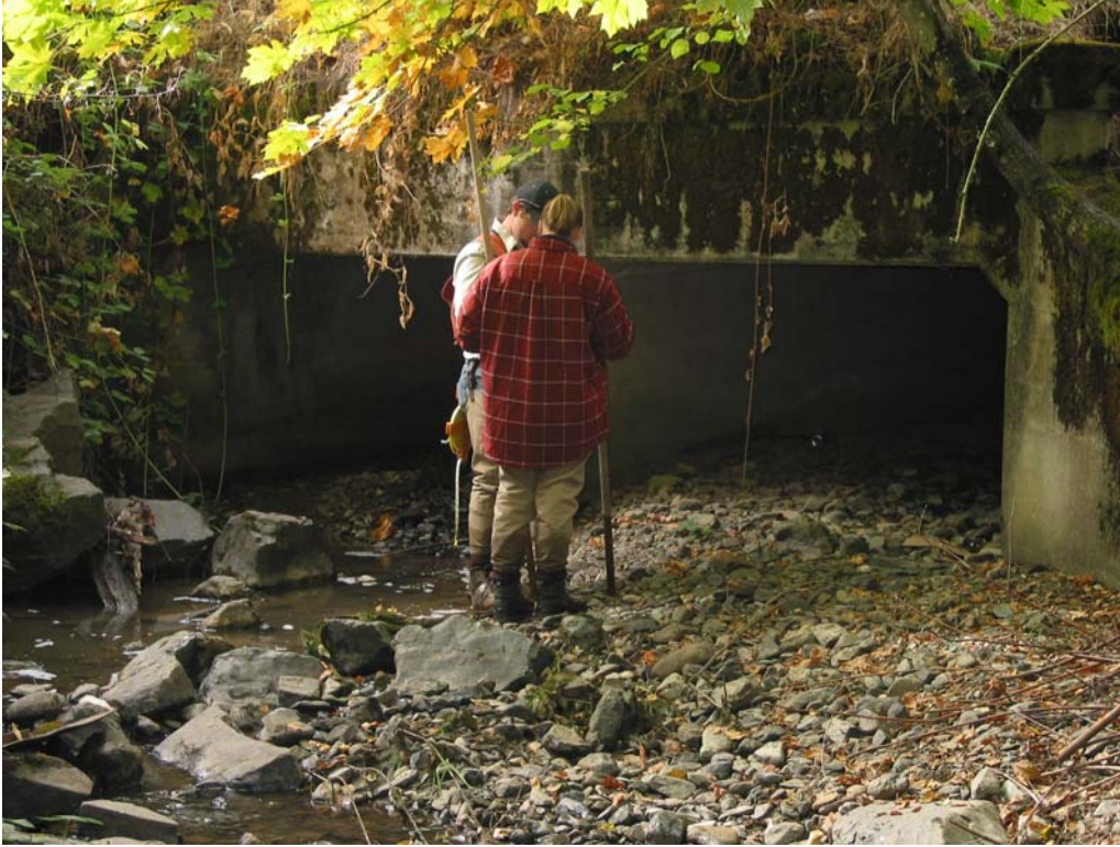
Figure 21. Culvert #1 outlet on Jordan Creek at I-5.
